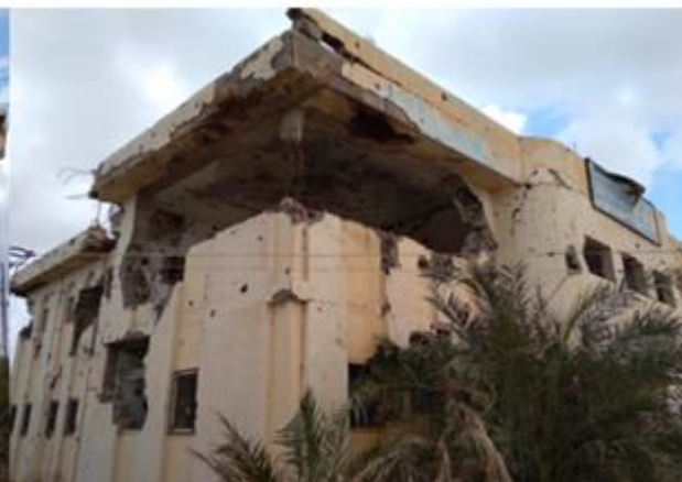
Photo 1.2 South elevation of the building
