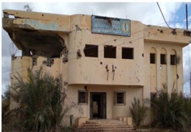
Photo 1.1 West-south elevation of the building
