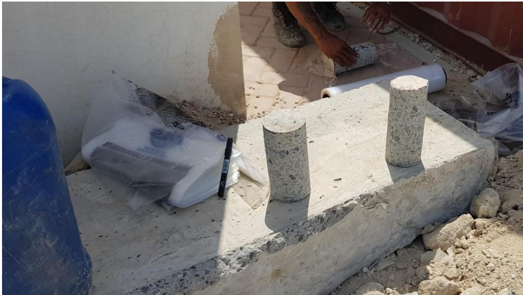
Figure 6 Coring and sealing of the core specimens.
