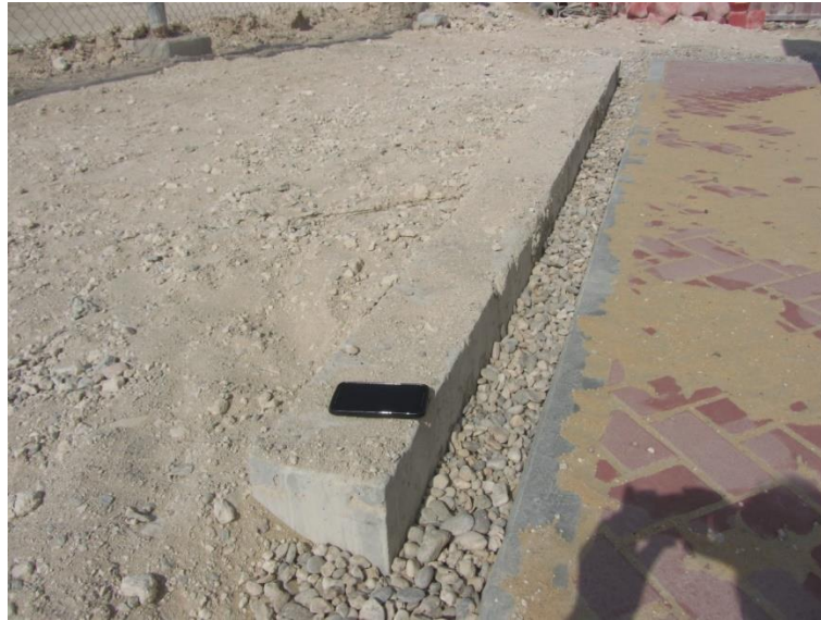
Figure 3 Additional beam cast for coring and long-term monitoring behind buildings.
