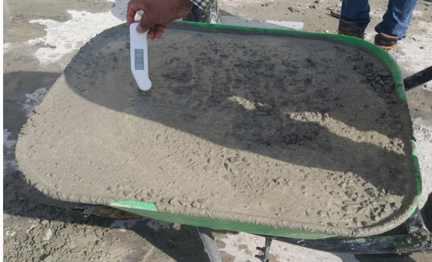
Figure 4 Measuring concrete temperature on site.
