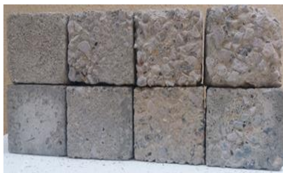
Figure 4 View of the studied specimens after the deicing salt test.
