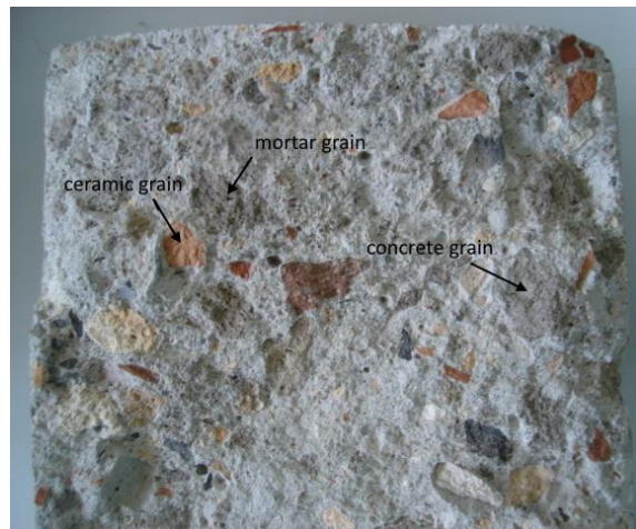
Figure 6 Fractured surfaces of concrete along with the recycled aggregate.
