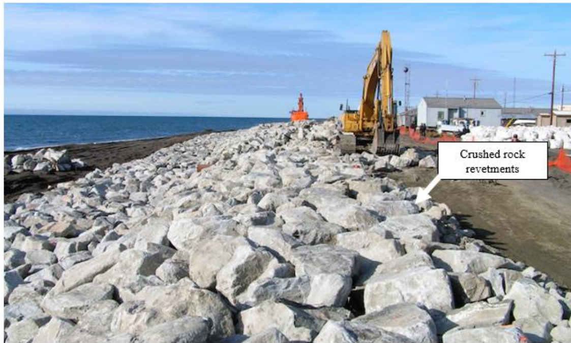
Figure 10 Rock revetments along the Alaskan Arctic coast (adapted from [43, 90]). Revetments show the fewest reported failures of any coastal-protection class and, unlike foundation strategies, can be retrofitted to existing shorelines-making them the most immediately deployable response to compound coastal hazards.
