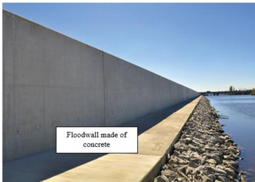
Figure 11 Floodwall along the coastline (adapted from [43, 91]). Identified by officials at 7 of 15 Arctic bases as a viable storm response, floodwalls exemplify low-maintenance accommodation measures that protect high-value waterfront assets without altering the structures themselves.
