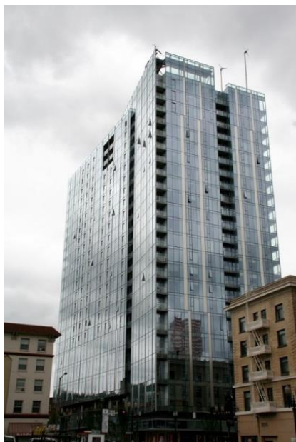
Figure 8 Twelve West building, Portland, USA [51], permission for use authorized by Wikimedia Commons.
